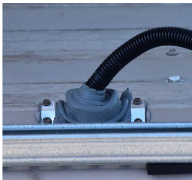
Figure 17: A Dektite* with a metal roof flashing
