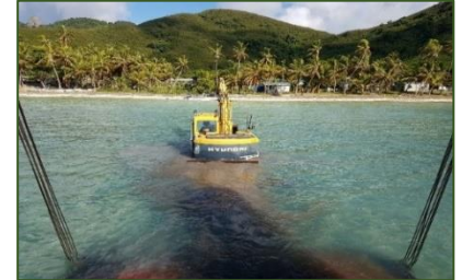
Fig. 3 Excavator carrying cargo to shore
