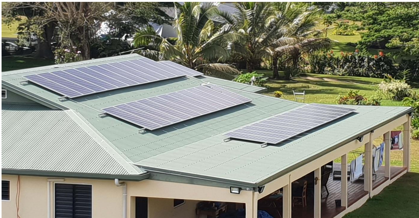
Caption: Off grid PV System installation in Port Villa.
