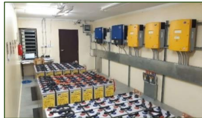
Fig. 2 SMA inverters, GNB storage, comms. System & solar switchboard room
