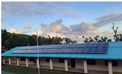
Fig. 1 Part of the 30kWp roof-mounted solar plant
