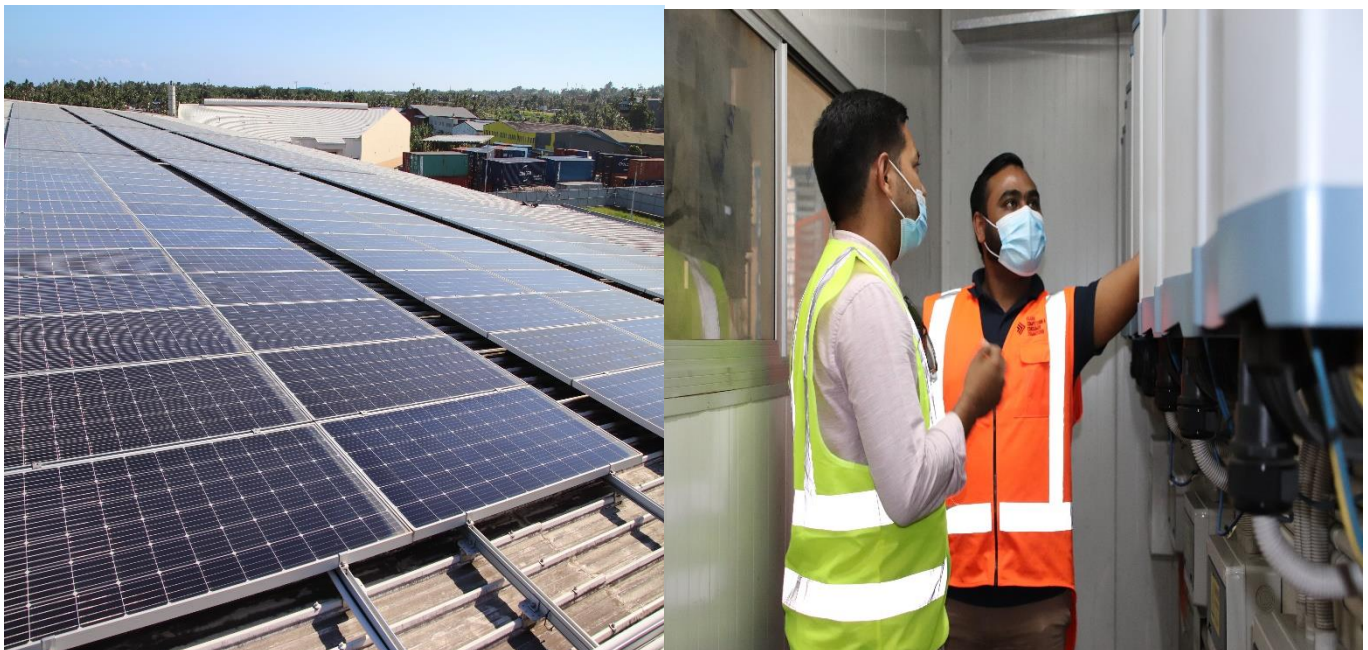
Caption: FCCC conducting inspection at one of the site
