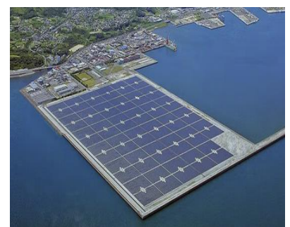
Kagoshima PV, Japan (Source: John Major, Univ of Liverpool)
