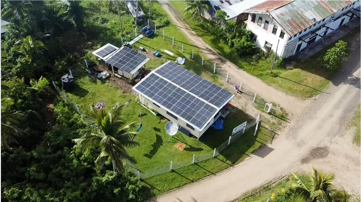
Off grid Solar Project on Rabi Island, Fiji
