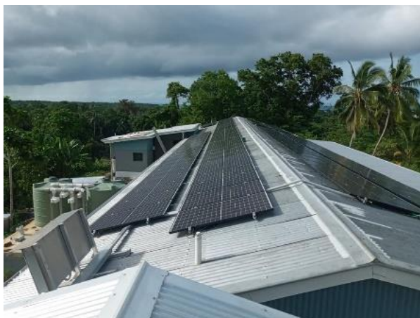
a) PV array for Aola System
