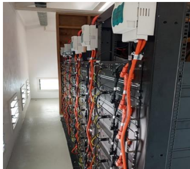
Caption: Battery racks of the Aola System
