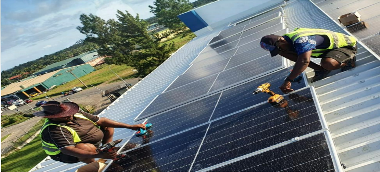
Nakasi (Fiji) Solar Project in Progress
