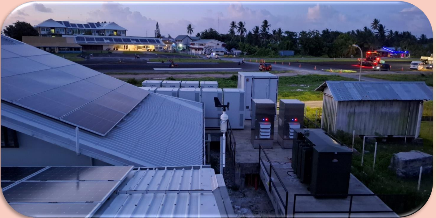
FUNAFUTI 3MW/3.35MWH BESS AT TEC POWERSTATION
