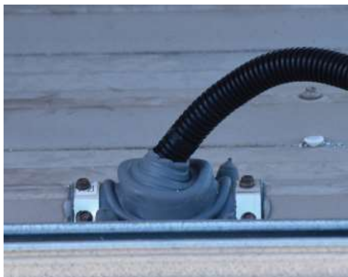
Figure 24: A Dectite® with a metal roof flashing
