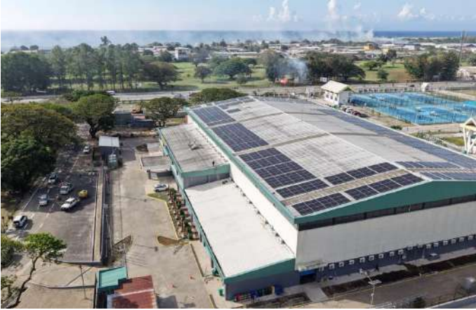
Friendship Hall 648 panels and 108 air conditioners
