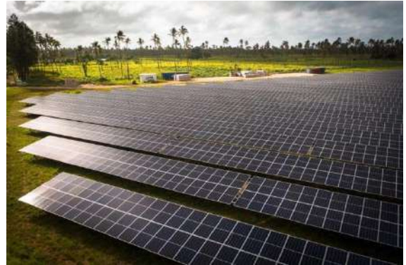
1MWp+1MWh BESS Taveuni
