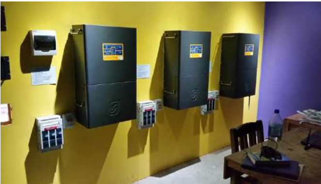
Air Terminal Services Building - Nadi Airport - 175kW Grid Connect system with Winaico and Enphase Microinverters
