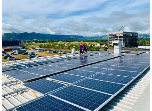
Air Terminal Services Building - Nadi Airport - 175kW Grid Connect system with Winaico and Enphase Microinverters
