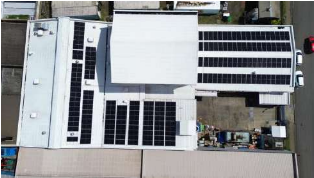
Narseys 90kW System
