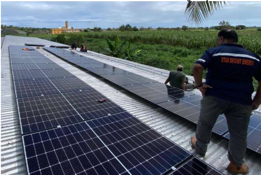
Western Eggs 15kW and 14.4kWh battery system Systems installed by SEIAPI member : Starbright- Fiji
