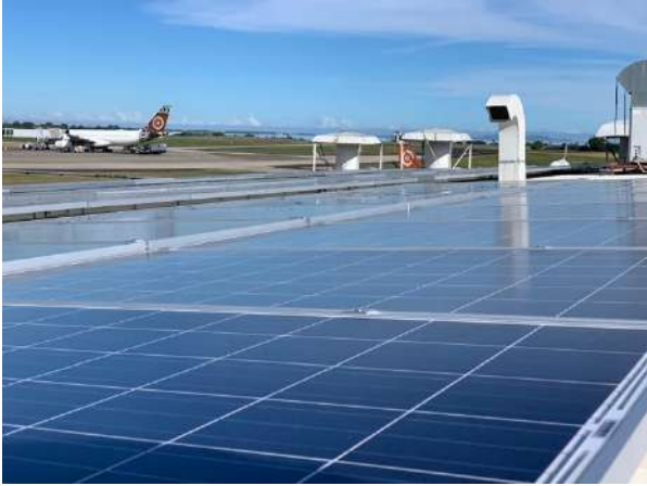
Air Terminal Services Building - Nadi Airport - 175kW Grid Connect system with Winaico and Enphase Microinverters
