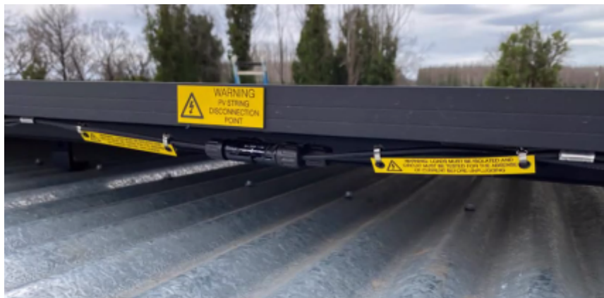
Figure 16 Example of a disconnection point
