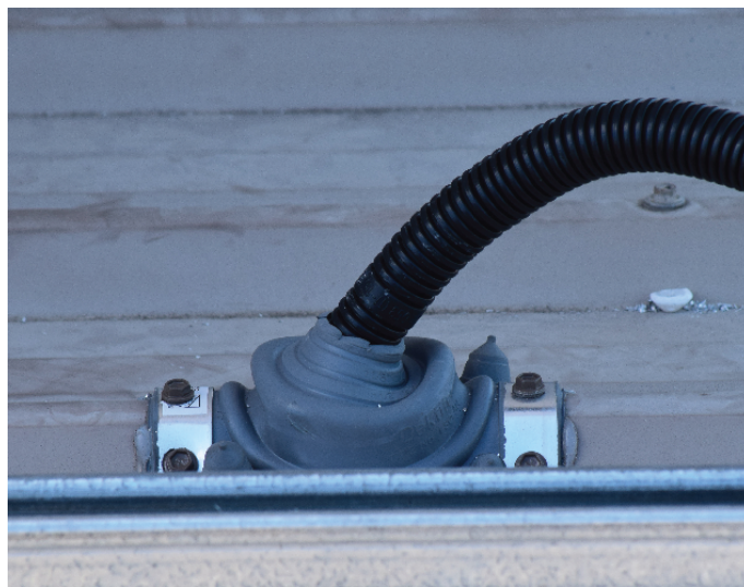
Figure 19: A Dektite® flashing on a metal roof.
