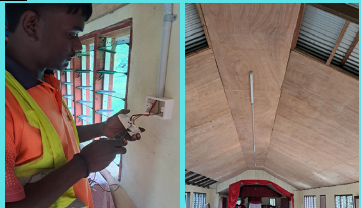
Caption: Island Solar (Fiji) Ltd working on the installations at Yadrana Village. Photo supplied by Island Solar (Fiji) Pte Ltd
